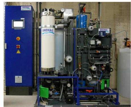
The installed ultrafiltration module is designed for a low flux, so that intervals between chemical cleanings of about 3-6 months can be achieved.
